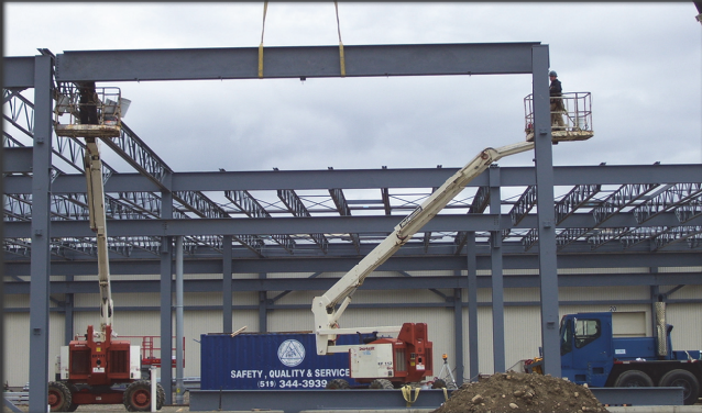
Chemical Plant: Complete Steel Fabrication, Painting and Erection
